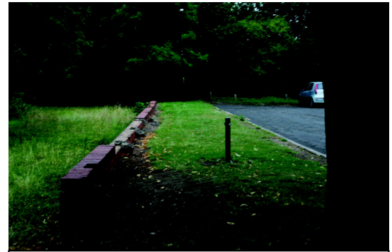
Perimeter wall along Swanslength
